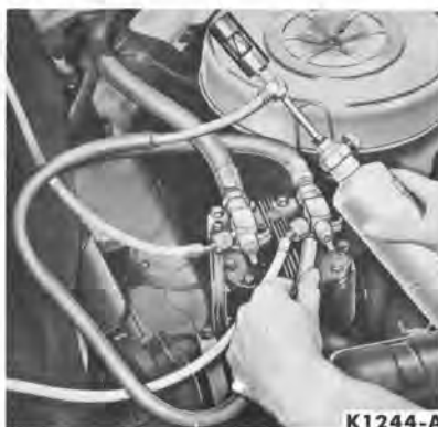
FIG. 14—Using Leak Detector
